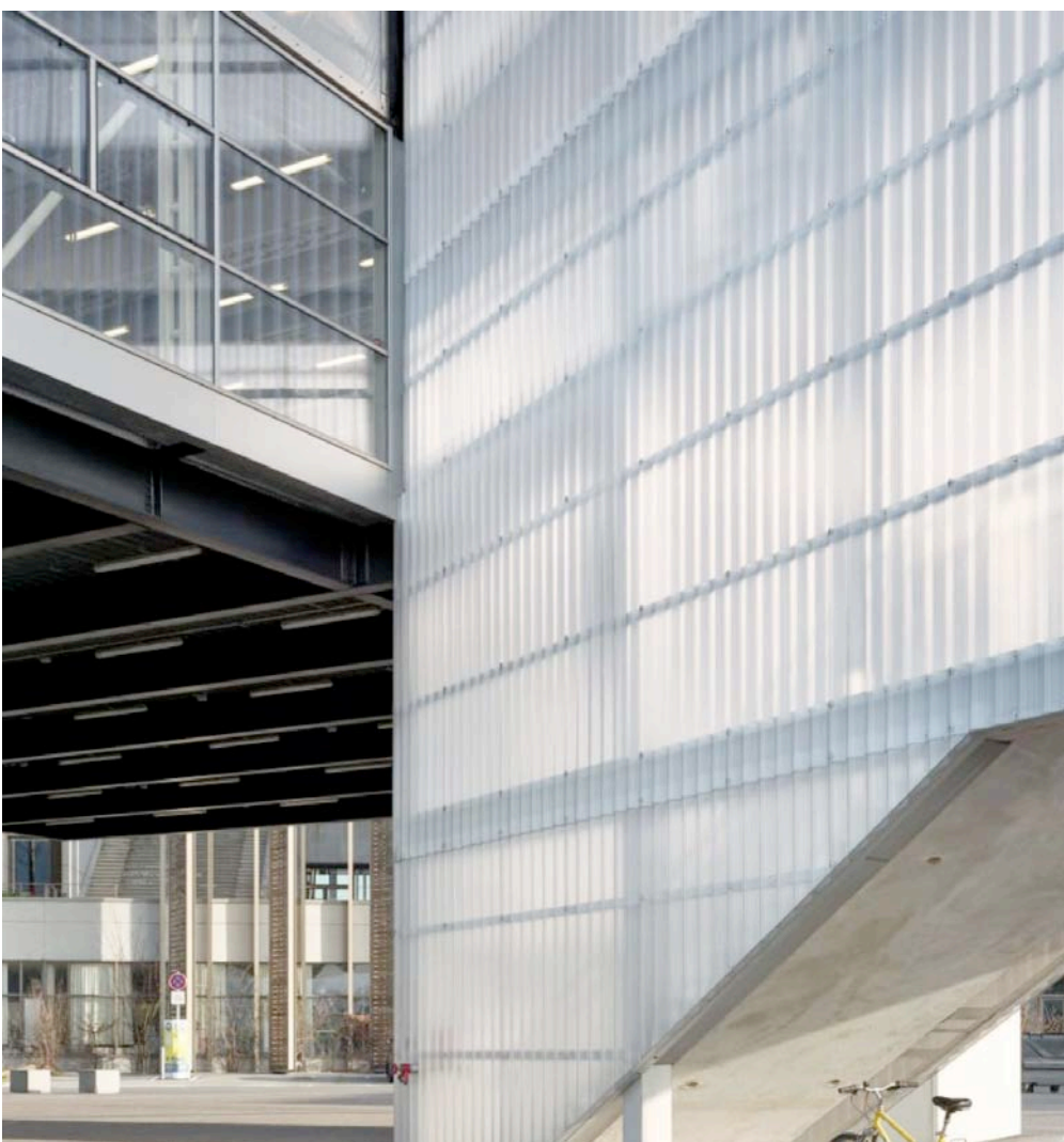
Reference fasády Research center in Caen, Bruther
